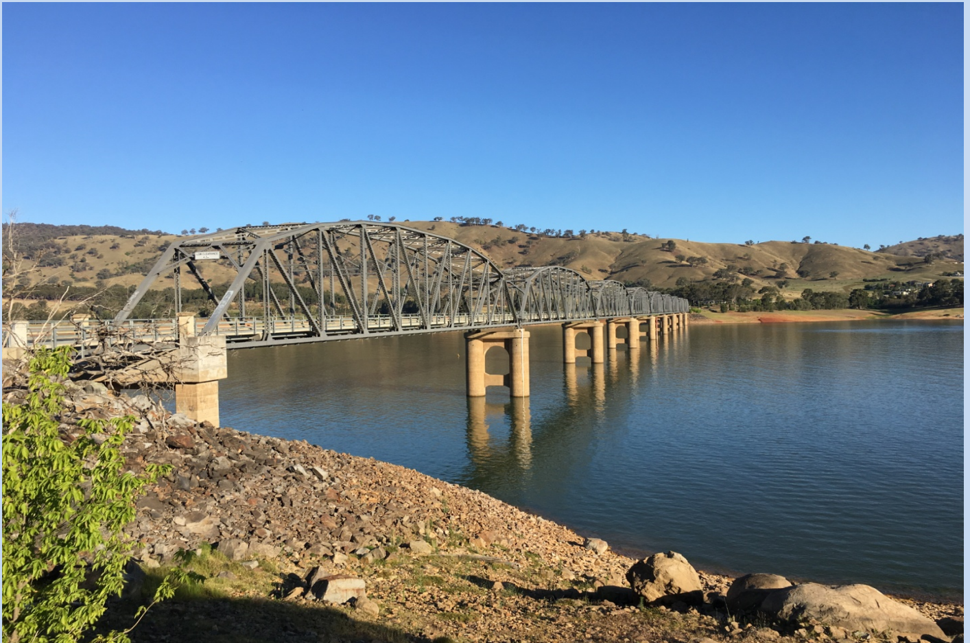
The Bethanga Bridge looking east towards Victoria from the NSW side of the Murray Arm of Lake Hume.
